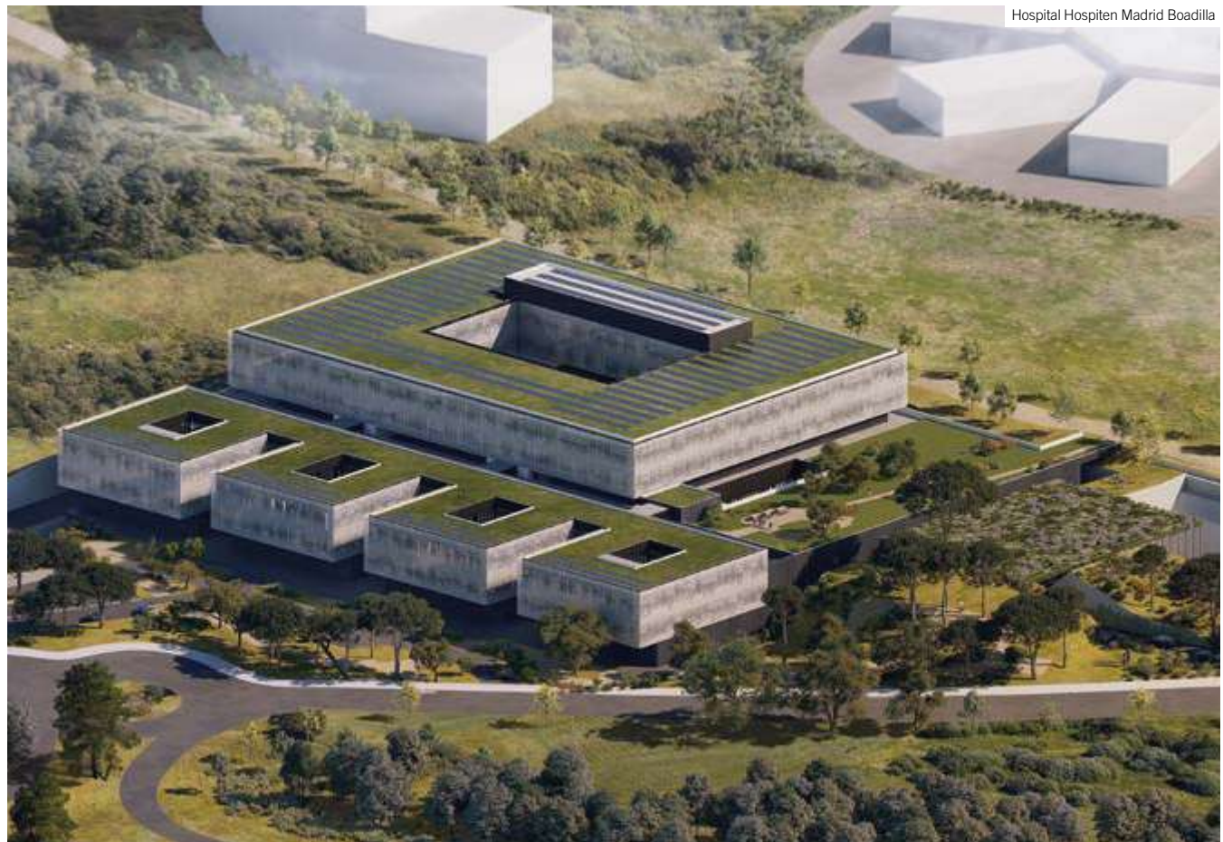
Hospital Hospiten Madrid Boadilla
