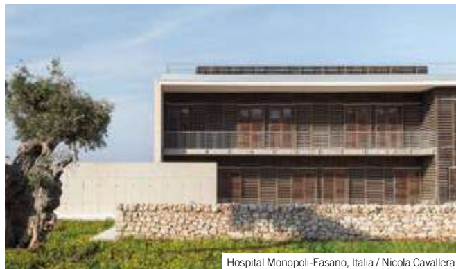
Hospital Monopoli-Fasano, Italia / Nicola Cavallera
